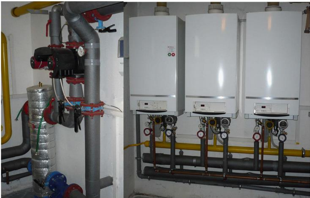
Fig. 2 Boiler room after construction in 2009
