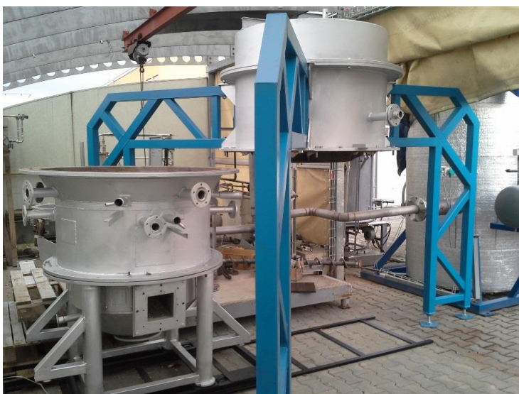
Fig. 3 Fixing of the upper part of the reactor on beams
