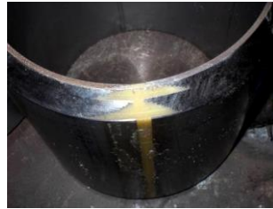
Fig. 2.5 Gap between the ends of roll bended strips after flooding by the two-component epoxy
