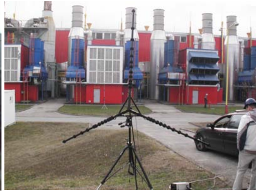
Fig. 6: The acoustic camera installed at measurement site
