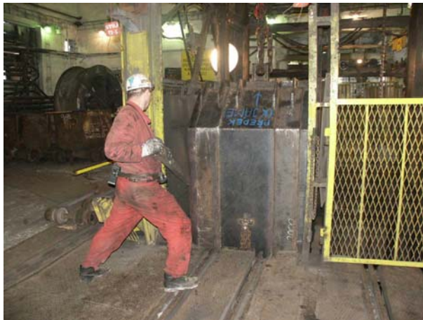
Fig. 8 Container lowering in shaft to adequate filling place
