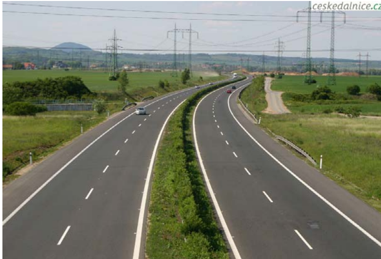
Fig. 1: Example of a section of a highway, central green lane without crash barriers.
